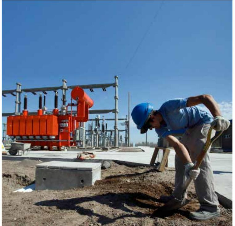
Construction of a new 132 kV Substation. The project will be built on an area of 10,000 square-meters, with two 132 KV input and output line hubs, two 132 KV bars (main and transfer), a transfer hub at 132 KV, and a transfer hub of 132/33/13.2 KV 30/30/30 MVA, 3 (three) 33 KV cells, and 6 (six) 13.2 KV cells.
