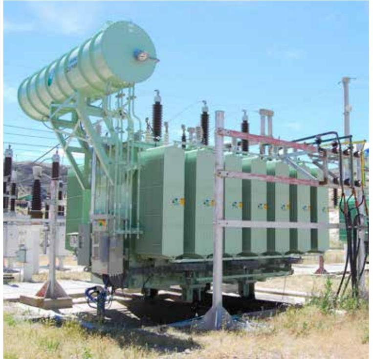
The project will involve the construction of a 132/33/13.2 KV substation at El Solito, including the installation of a 15 MVA transformer at 13.2 KV. At General Conesa, a 132/33/13.2 KV substation will be built with a 30 MVA transformer at 13.2 KV.
