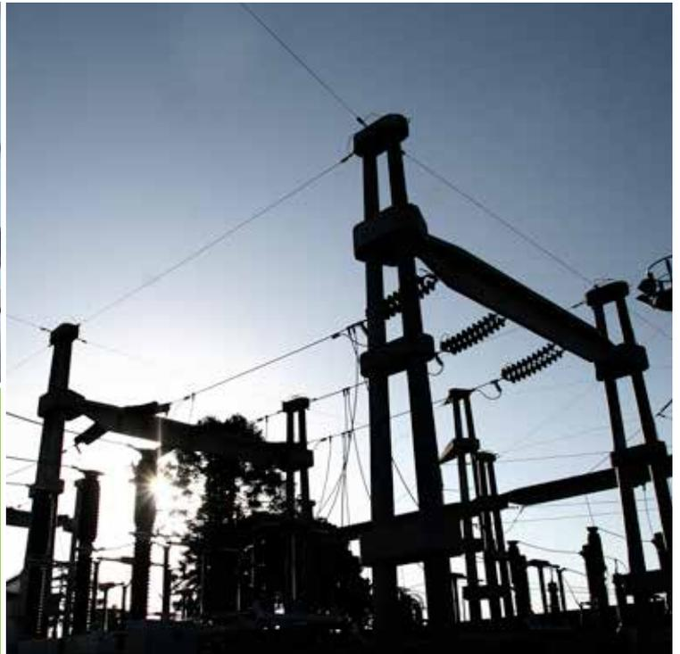
The project embraces the construction of a full Substation on a 1-hectare area, 2 (two) 132 kV line hubs, 1 (one) 132/33/13,2 kV - 15/10/15 MVA transformer with 132 and 13.2 kV equipped fields, building, etc.
